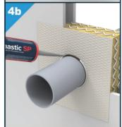
Seal the remaining recess with Multimastic SP or with the Multimastic C System or Multimortar System.
