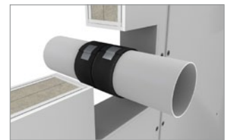
Fixing of the finished wrappings with duct tape
