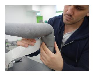
**STEP 5**If required use Tubolit tape or clips to secure any joins.
