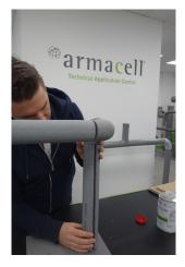
**STEP 4**Fit the cut Tubolit to the Tubolit Quick fittings.
