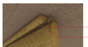
50mm Fire Barrier compressed between soffit and clamping plate at max 450mm centres
