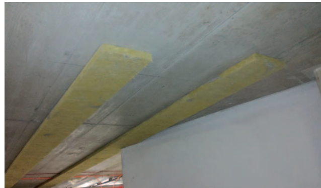
Fig. 18 Semifinished fire protective cladding ORDEXAL® KARBON ALB without final surface layer
