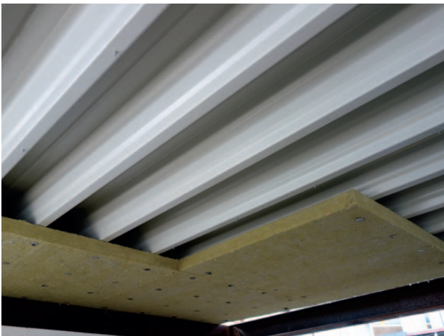
Fig. 9 System ISOVER FireProtect® for fire protection of corrugated steel is characterized by light weight and small height, but also a direct fixing to the corrugated steel without need of help of suspension construction
