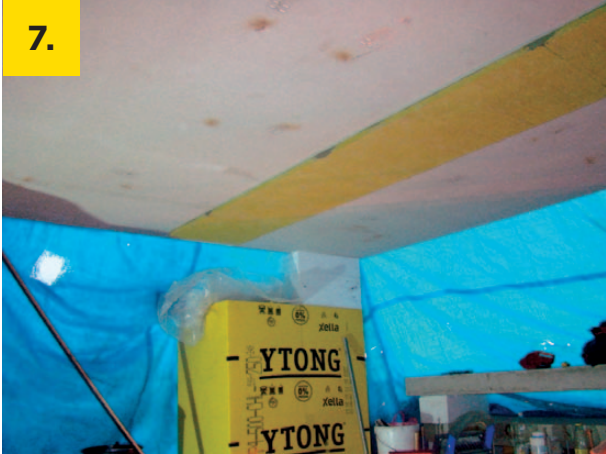
7. Installation of the first row of slabs - inspect the straightness of the row
