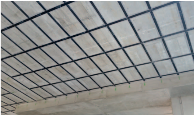
Fig. 17 Carbon fiber reinforced lamellas before fire protection
