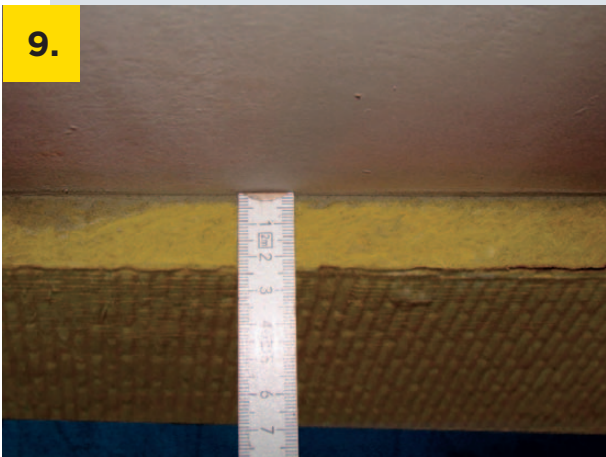
9. Check the system thickness, 20 mm slab, 3-4 mm layer of adhesive
