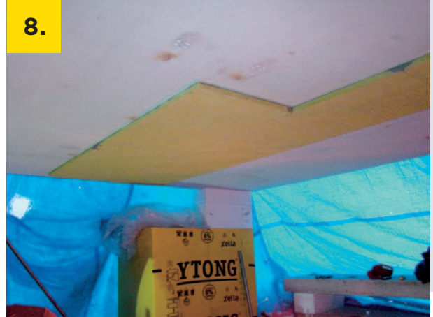
8. Install other slabs by pressing them against the edge of the already installed slabs (the edges are not glued)
