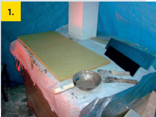
Inspect the slab and the tools used
