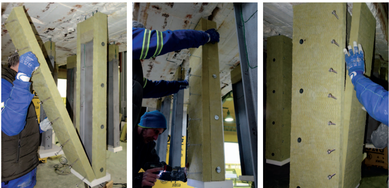
Fig. 5 Both methods can be also combined – important is to keep the distances (between pins 300 mm and between Fire Screws 150 mm)
