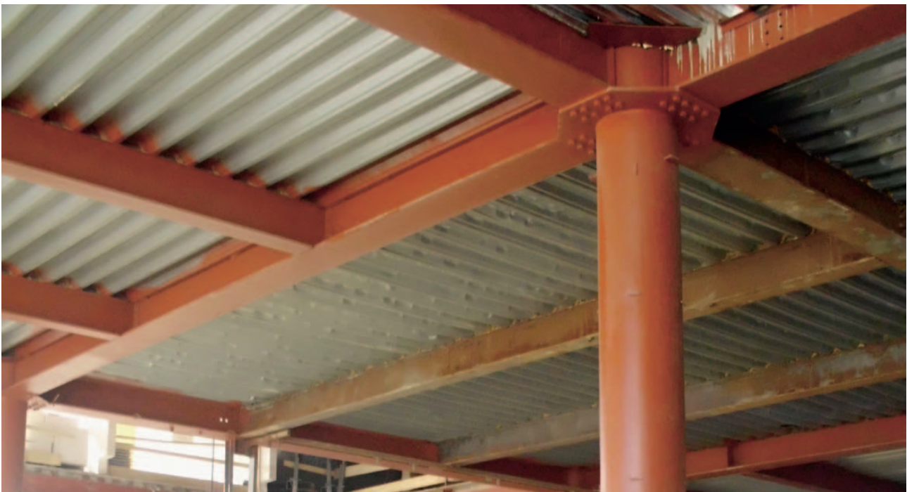
Fig. 17 If the reinforcement is placed in the trapezoidal sheet waves, a ribbed ceiling with a bearing "T-section" will be formed and therefore a statically optimal use of the height of the concrete slab will be achieved. When establishing the insulation capacity criterion I, you can consider the height h_1 or the so-called effective height of h_{eff} ; the thickness of the distribution layers h_f can also be included in I criterion in individual cases.
