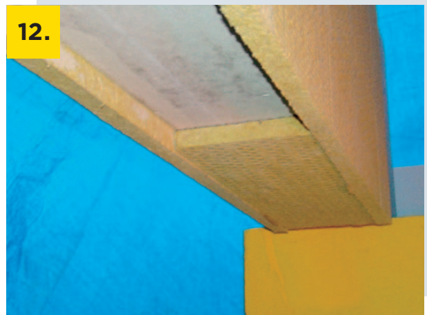
12. The flange is glued in the end
