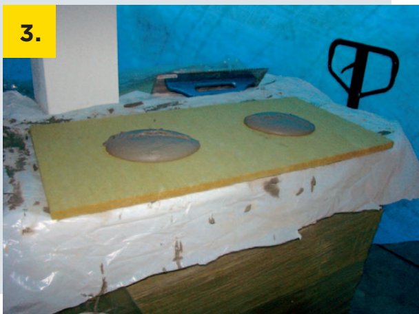
Apply an adequate amount of the adhesive on the slab
