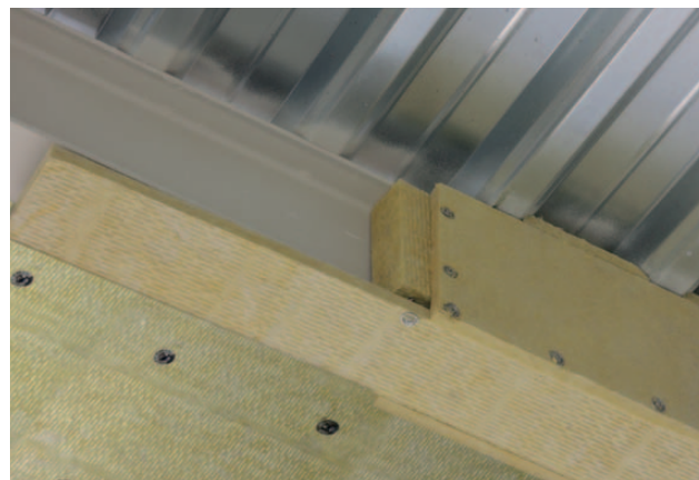
Fig. 14 The four side fire protection of a steel beam (using the ISOVER FireProtect® 150 slabs to backfill a trapezoidal profile)
