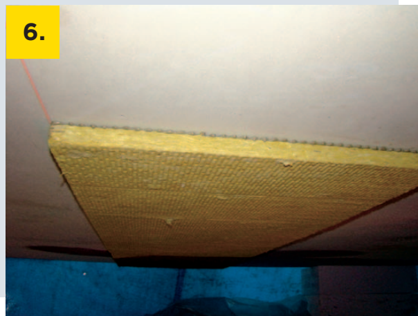
Check the bonding over the entire surface - Dexaflamm B adhesive is slightly pushed out and visible
