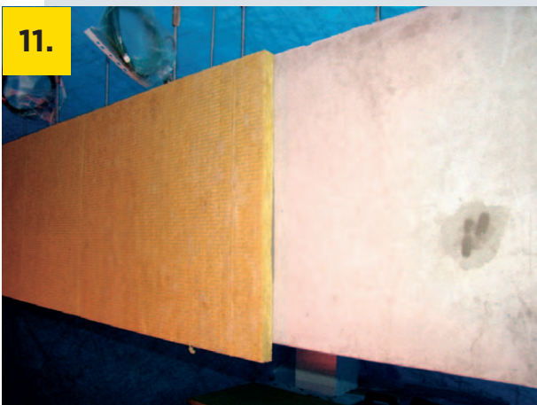
11. In case of a beam, the sides are glued first
