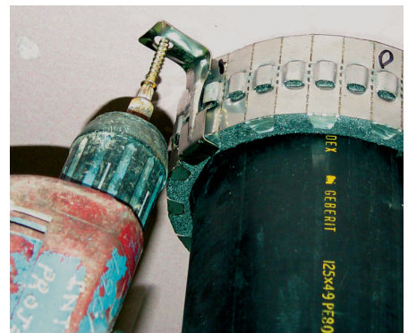
Step 6 - Secure collar in place
