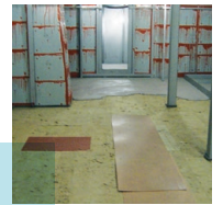
ROCKWOOL A-60 floating floor system (example)
