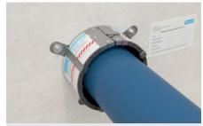
8. Fix the collar with M6 or M8 threaded rods (light partition walls), for rigid walls and floors use concrete screws (Ø 6 mm, I = 50 mm) or anchors.
