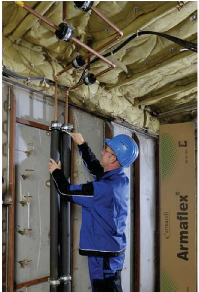
Figure 5: Installing Armafix pipe supports
