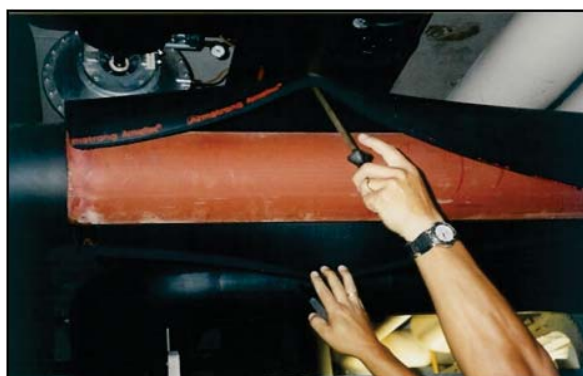
AF/Armaflex insulation inspected after 20 years with \mu and \lambda values preserved
