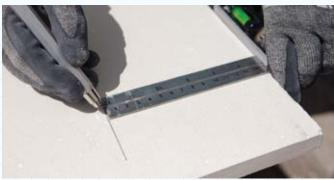
3 Cut Flange Panel – Cut boards using a hand saw with hardened teeth or a power circular saw in conjunction with tungsten carbide tipped blades, or a jigsaw. All cutting should be carried out in well ventilated spaces, using dust extractors. Operators should wear protective face masks.
