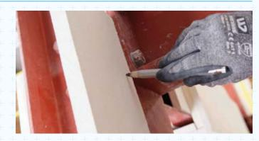
5 Measure for Web Panel – Measure the web of structural steel column plus the thickness of the VERMICULUX®-S flange panel. (20, 25, 30, 35, 40 or 50mm).
