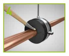
Before insulating the pipe, glue the edges of the pipe support to the pipe.
