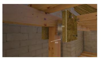
25mm thick ROCKWOOL BeamClad<sup>®</sup> fixed with Firepro Glue and nailed, or 50mm Fire Barrier secured with screws and large square washers. Use 50mm nails for BeamClad<sup>®</sup> and 70mm screws for Fire Barrier.
