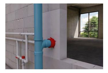
Firestop Compound is a specially formulated gypsum-based compound, which is mixed with water to be trowelled or poured around service penetrations.
