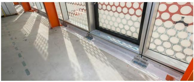
SoftSeal installed as a linear joint seal
