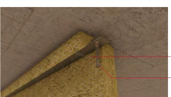
50mm Fire Barrier compressed between soffit and clamping plate at max 450mm centres
