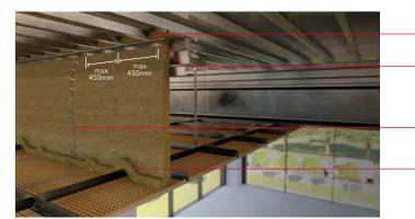
Fire Barrier cut and pushed up into profile as fire stopping
