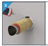
Apply Multimastic SP generously in the gap to prevent air bubbles.
