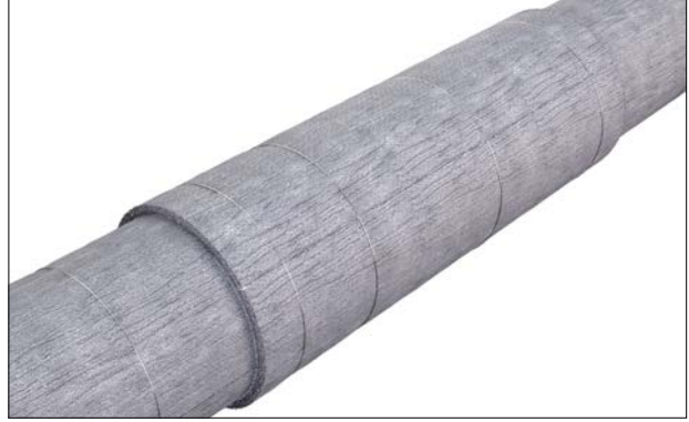
Figure 14: Securement of ArmaGel with stainless steel wires.
