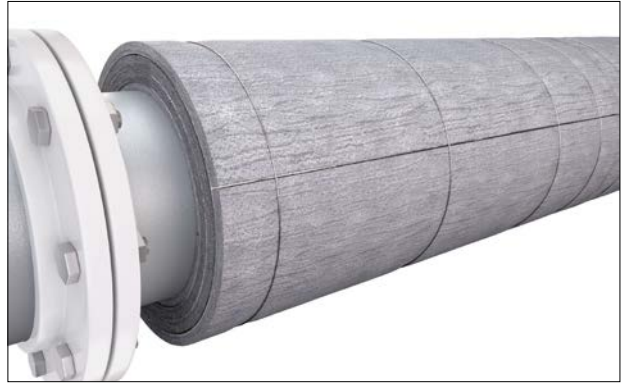
Figure 24: Positioning of final layer.
