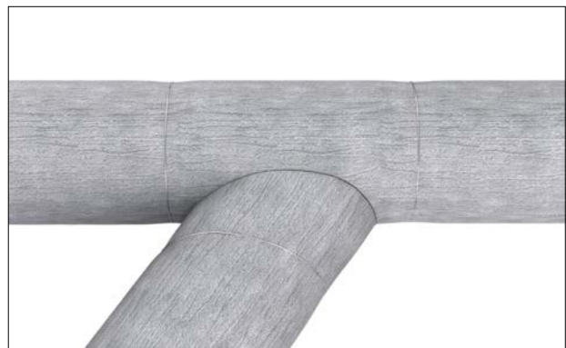
Figure 55: Completed tee cover.
