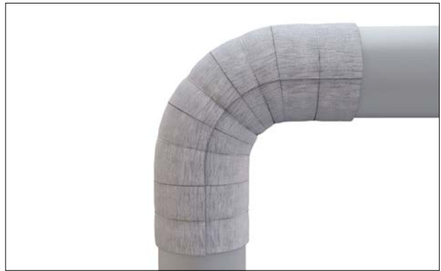
Figure 37: Completion of segment installation.
