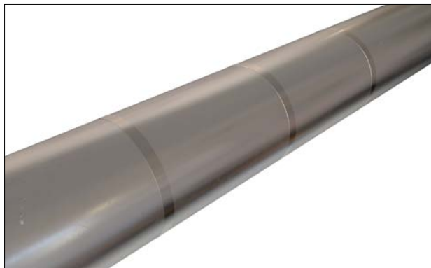
Figure 27: Completed metal jacketing.
