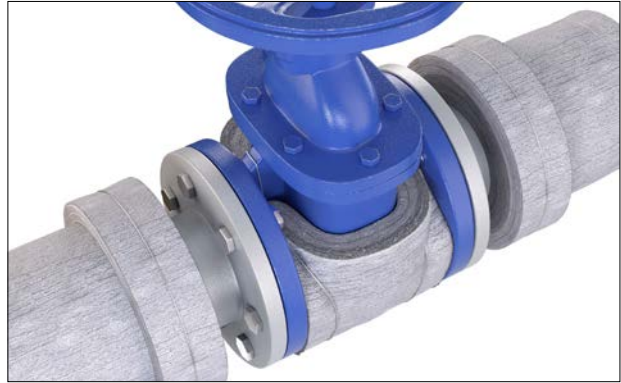
Figure 59: Packing out of air-space.
